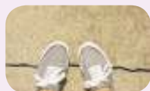
7. stepping on a crack
