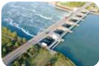
Rance Tidal Power Station, France
