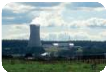
The Ohaaki Geothermal Power Station, New Zealand
